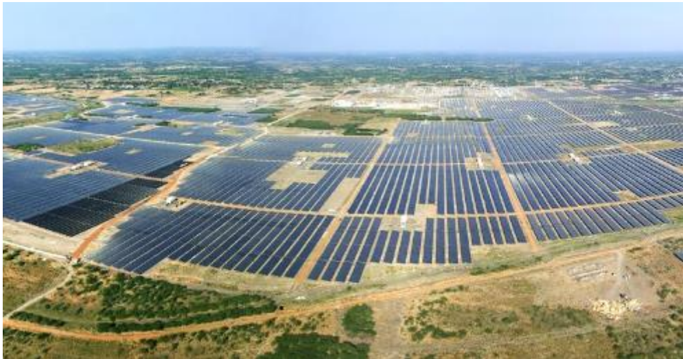
Figure 4: Kamuthi Solar Farm
